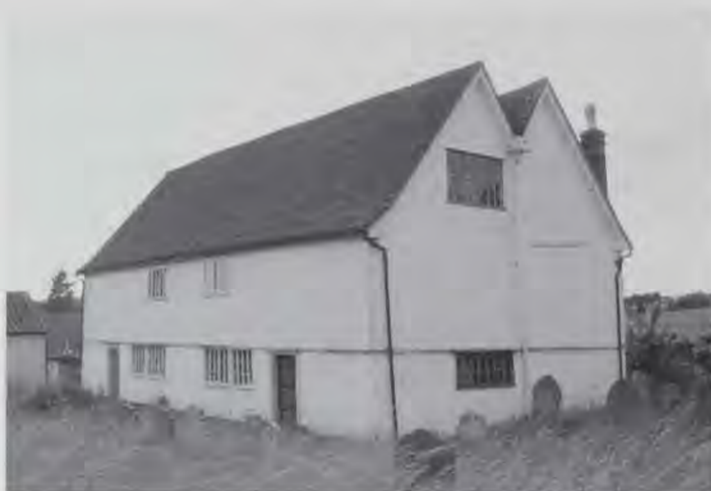
2 Walpole, Suffolk. Exterior of the Walpole chapel, converted to a meeting-house in the late seventeenth century – once a timber-framed farmhouse.
