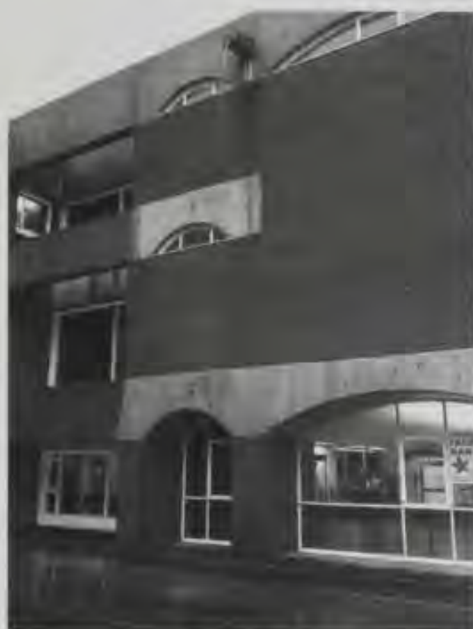
Fig 13 Water spout, Falmer House, Sussex University, shown channelling rain water from the roof to the interior moat.
